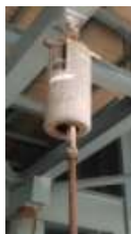
Fig 4.1 Variable load hanger
